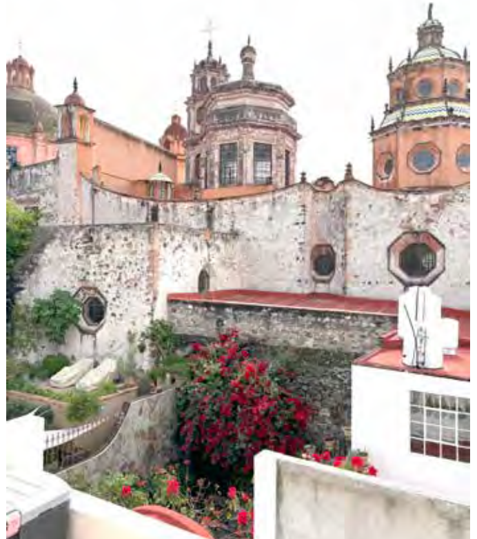
Rooftop view from the house
